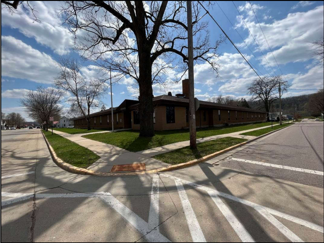
View looking southwest
