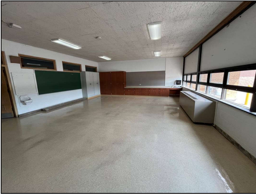
Typical classroom finishes (note the sink and drinking fountain)
