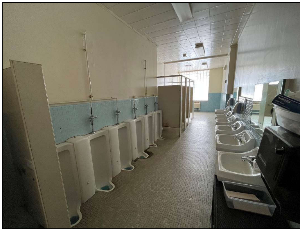
View of the restroom finishes
