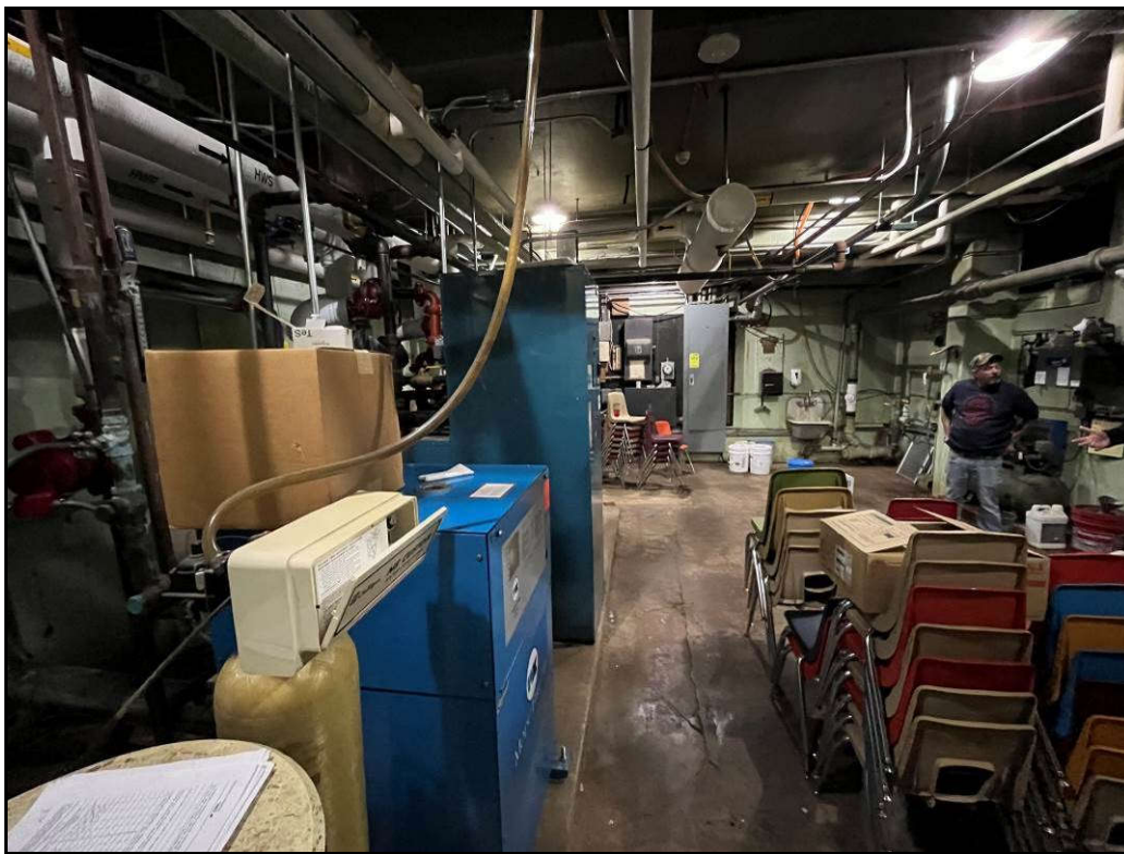
View of the basement
